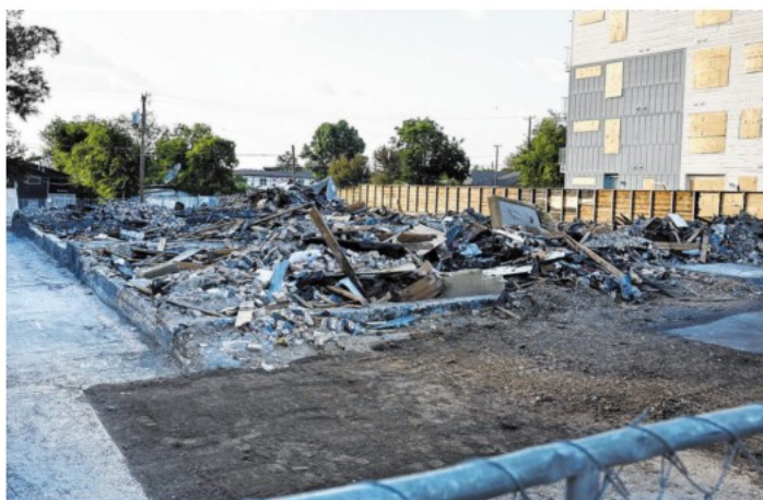
Debris from a deadly explosion and fire at The Clyde apartment building can be seen behind a fence in Oak Cliff on June 3 in Dallas. Three people were killed in the May 28 explosion and fire at the apartment building.
